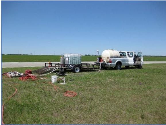
Mobile in-situ remediation equipment is staged to perform passive injections. Substances such as lactate or vegetable oil are inserted into the subsurface, where they act as a stimulating food source for naturally-occurring microbes. The equipment helps to implement a sustainable approach to efficiently remediate sites at Moody AFB.
