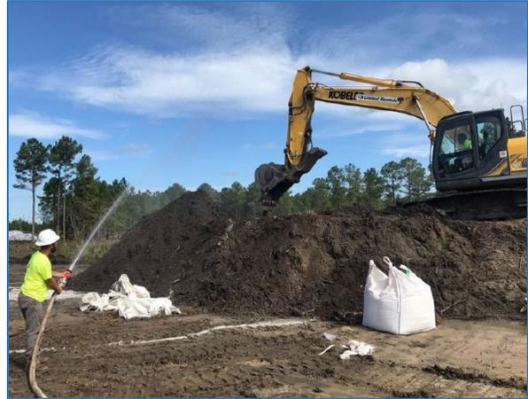
Soil stockpile being sprayed with water as it is being mixed with a powdered lead stabilizer (EnviroBlend®). This limited the EnviroBlend® from escaping into the air during the mixing process. Using the lead stabilizer allowed the soils to be disposed of as non-hazardous waste, saving \$1.5M on disposal costs.
