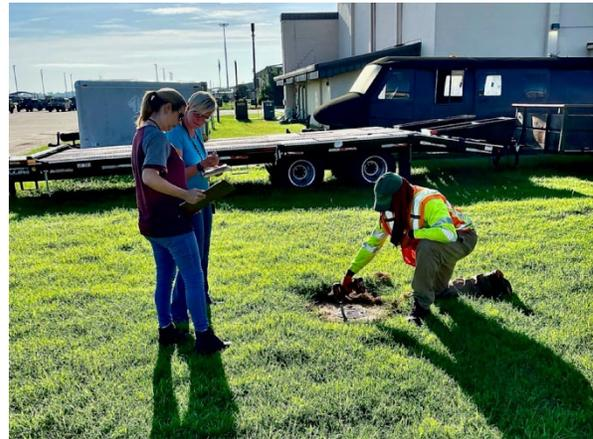
Georgia Environmental Protection Division (GA EPD) conducted a Corrective Action Permit Inspection in August 2021. All active remediation wells and systems were inspected to ensure compliance with permit requirements.
